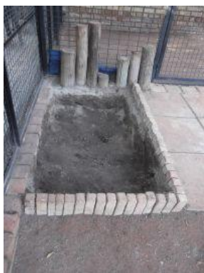
Photo 53: The sandpit when all the sand is removed
